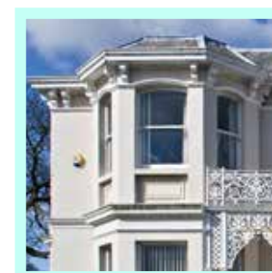
One over one pane sliding sash windows
