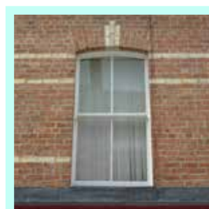
Quarter pane sliding sash windows
